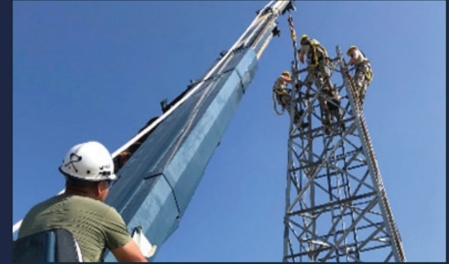
Weaver is an AFWERX innovation effort with the 364th TRS Cable & Antenna Systems Initial Skills Course. The 364th estimates Weaver will double or triple hands-on practice time.
